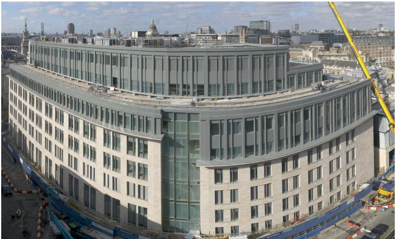
The new facility being built at St Bartholomew's Hospital in Farringdon.
