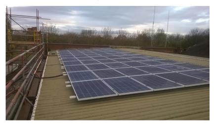
This project undertaken in 2016 involved the installation of photo voltaic cells to the main garage roof providing 15KW of power generation connected to the incoming electricity supply via metering located in the LV Switch Room. It was anticipated that the saving to the Trust will be £3,385.00 per annum on this site (based on current unit/hour rates).
