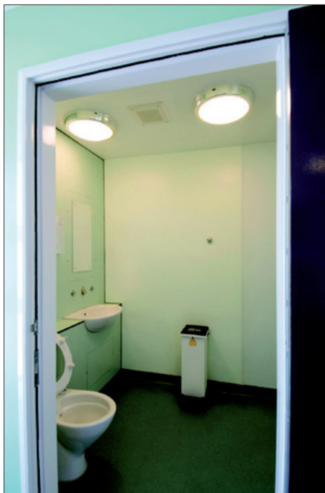
All fixtures and fittings should be anti-ligature
