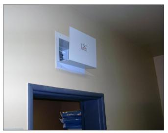
discharged through the pressure stabiliser may be used to offset the volume of supply air to the operating theatre.
