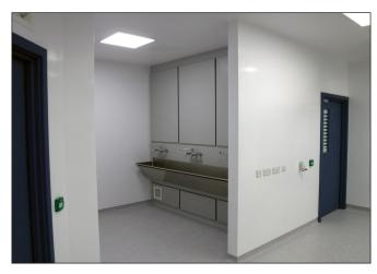
**8.46** Where the scrub is a trough on the wall or in an open bay within the operating theatre, it should have low-level extract under it.
