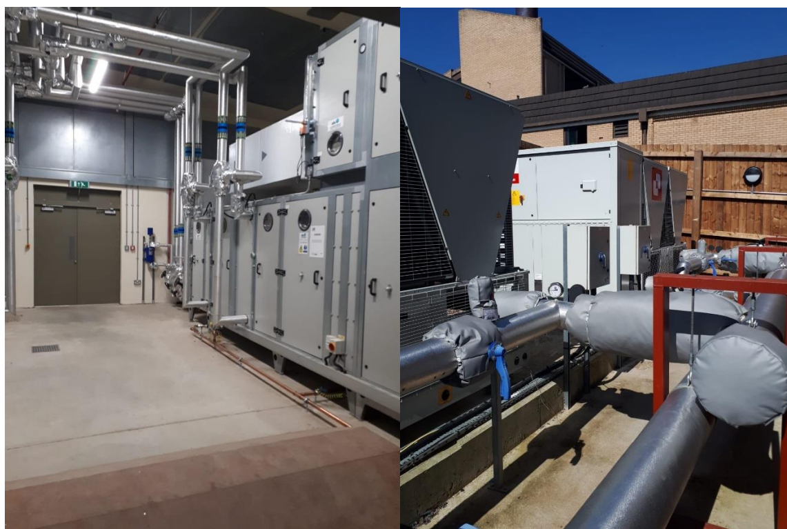
New ventilation and chiller plant at Dewsbury Hospital.
