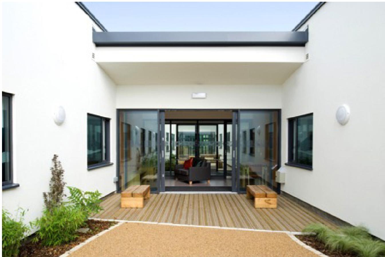
Sheltered outside space. Ferndene CYP (40 beds incl Low Secure), Cumbria Northumberland Tyne & Wear NHS FT, Laing O'Rourke, Medical Architecture
